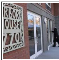
Arbor House in the Bronx Provides a Green Community for Low - Income Residents
